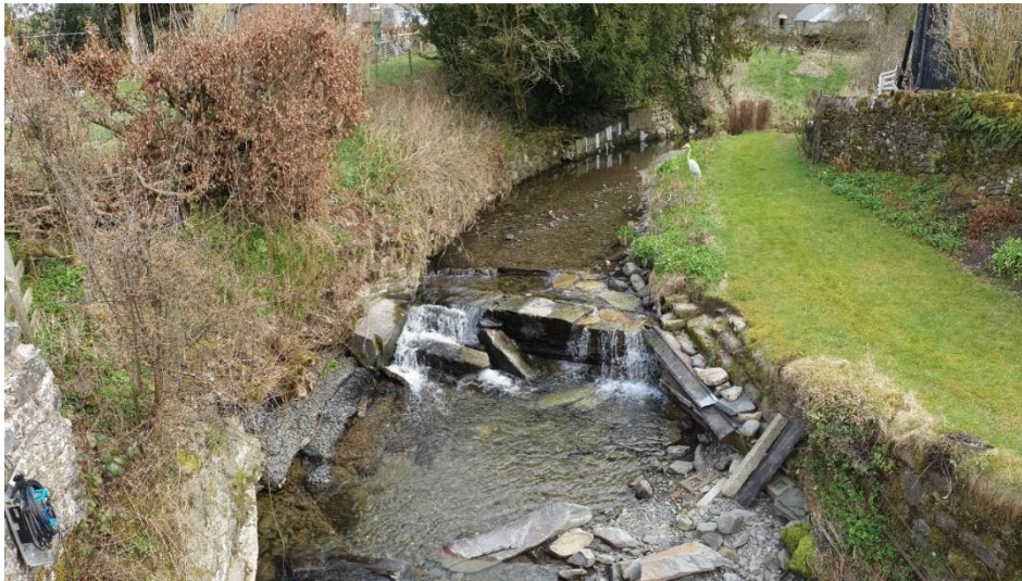
The small weir prior to removal. A large scour hole had formed immediately downstream of the weir.
