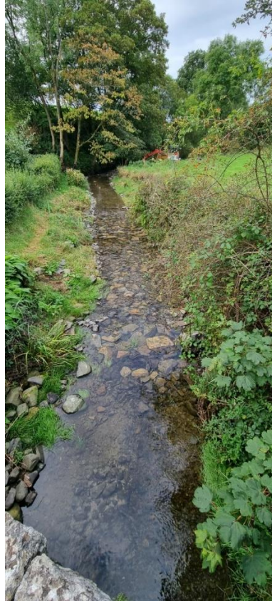
L: New regraded channel with the weir removed
