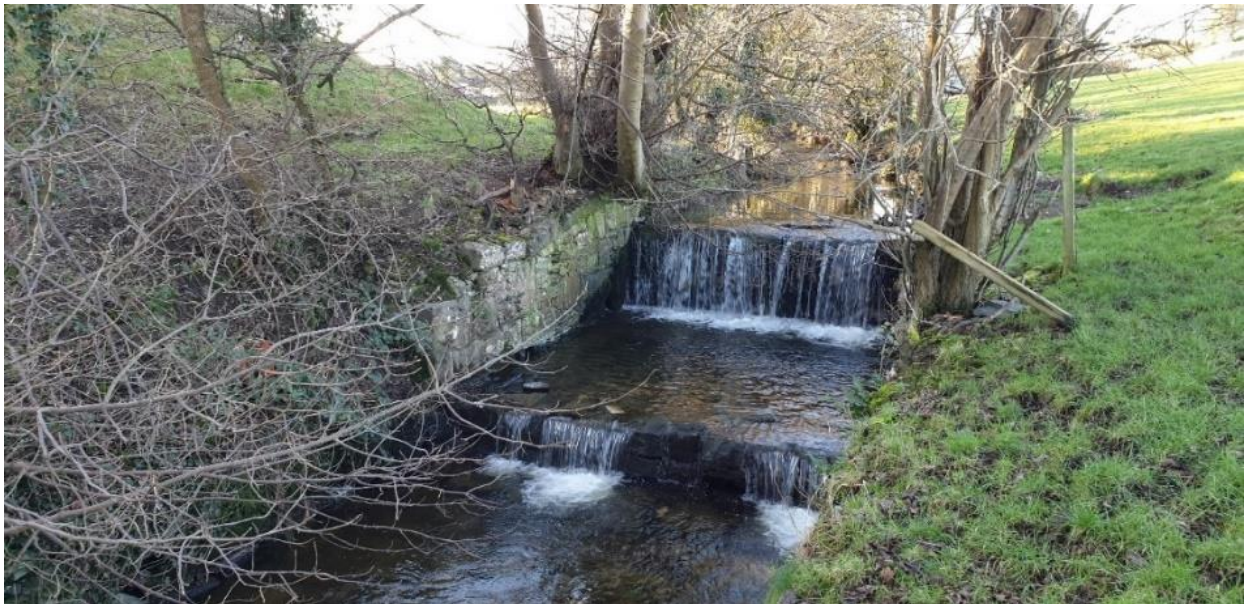
This is a double weir; the upper step is 1.4m high. The lower step is 40cms high
