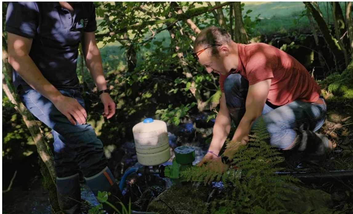
Installing a hydraulic ram pump SCRT/LIFE R4ever Kent/Mark Battista
